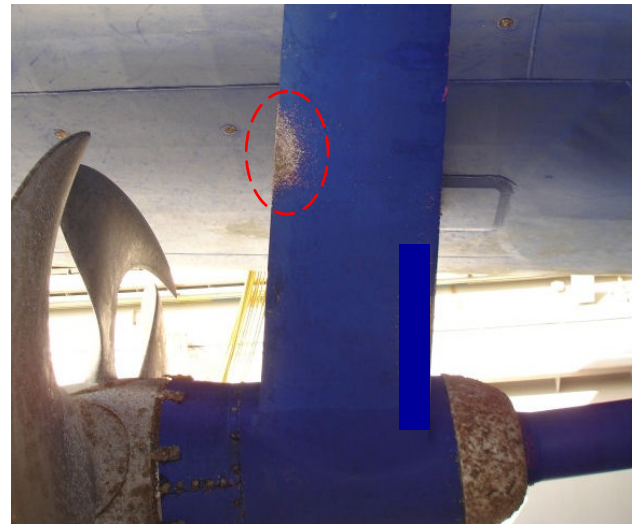
Figure 3: Cavitation damage on an A-bracket
