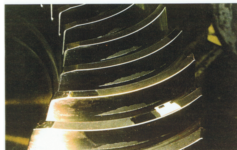
Figure 4. Picture of scuffing damage on six teeth of a crown wheel of diameter 1060 mm.
